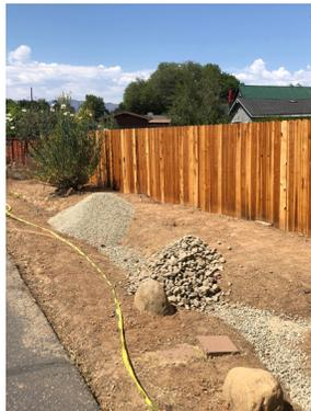
Photo 3: Gravel layers placed in trench.
