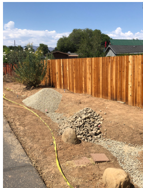
Photo 3: Gravel layers placed in trench.
